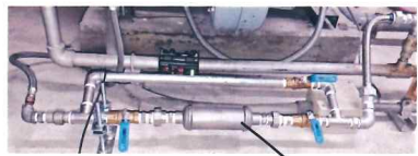
Attach to fuel supply piping. Super ball filter
